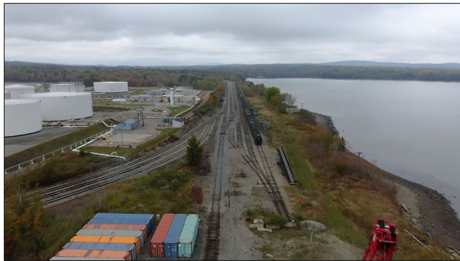
This photo shows Mack Point Terminal at Searsport. The Project calls for building two additional tracks to the right (south) of the southmost track with the tank cars on it. The track with the tank cars will be upgraded.
